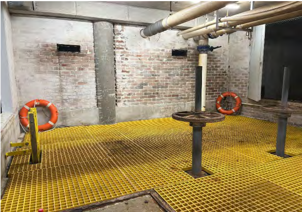
Figure 19 Seawater pit and valves in the basement
